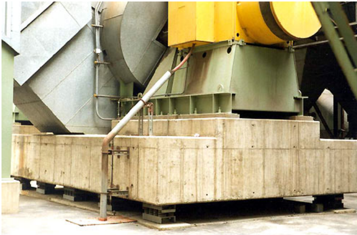
Vibration isolation of a fan
