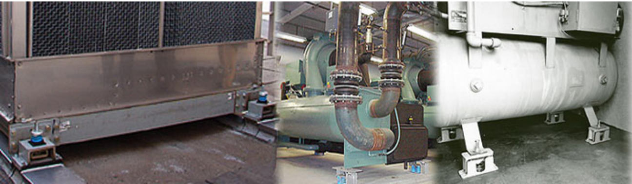
Vibration isolation mount
